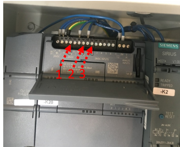
Figure 9: Snap shot of the CMU control box with focus on the external run connections
